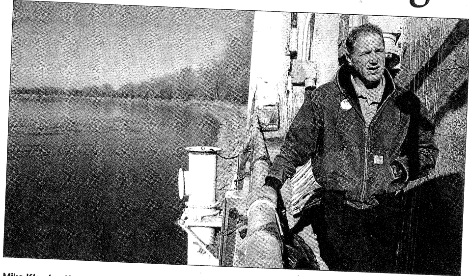
Mike Klender, Kansas City water supply division assistant manager for operations, stands by one of the city's auxiliary water intakes along the Missouri River in Kansas City, Mo., on Thursday. The Missouri is slowing sinking, as the river bottom erodes, which puts bridges at risk.
